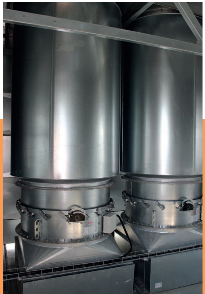
The exhaust fans are mounted directly on the exhaust air plenum in a closed cabinet protecting the fans against all weather conditions, as well as ensuring
