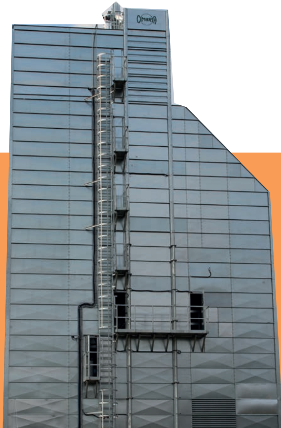
Inspection platforms placed at approx. 2.5 m intervals make inspection and cleaning easy.
